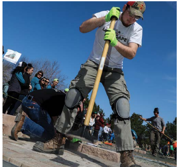
Matt Collingbourne in the hardscape installation competition.
