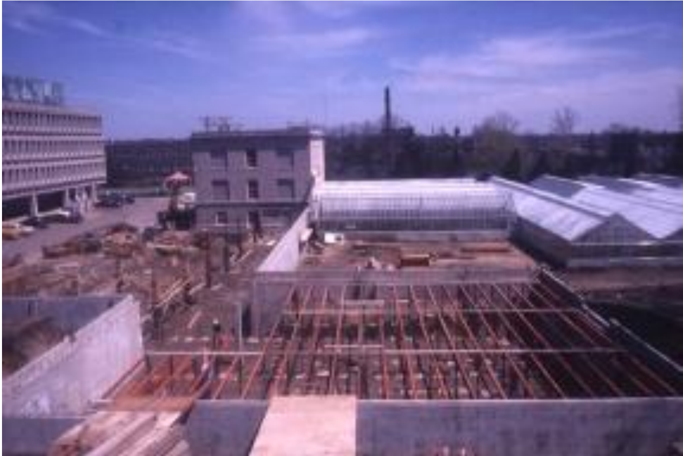
Construction of the ground floor.
