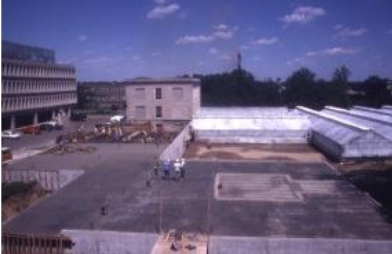
Preparing for construction of the first floor.
