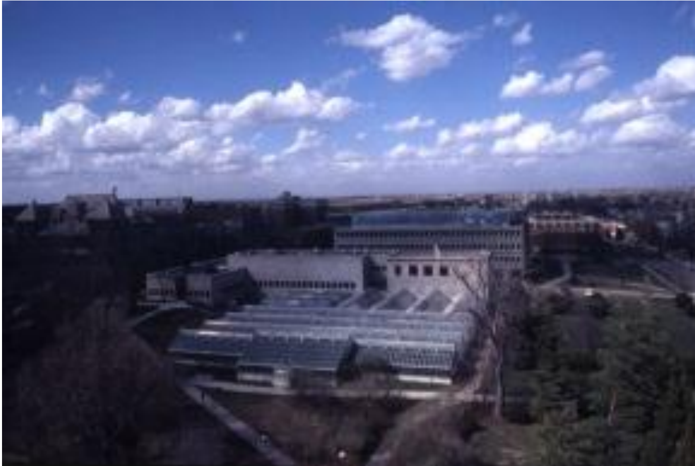
The finished addition and greenhouse complex viewed from Ross Hall looking north.
