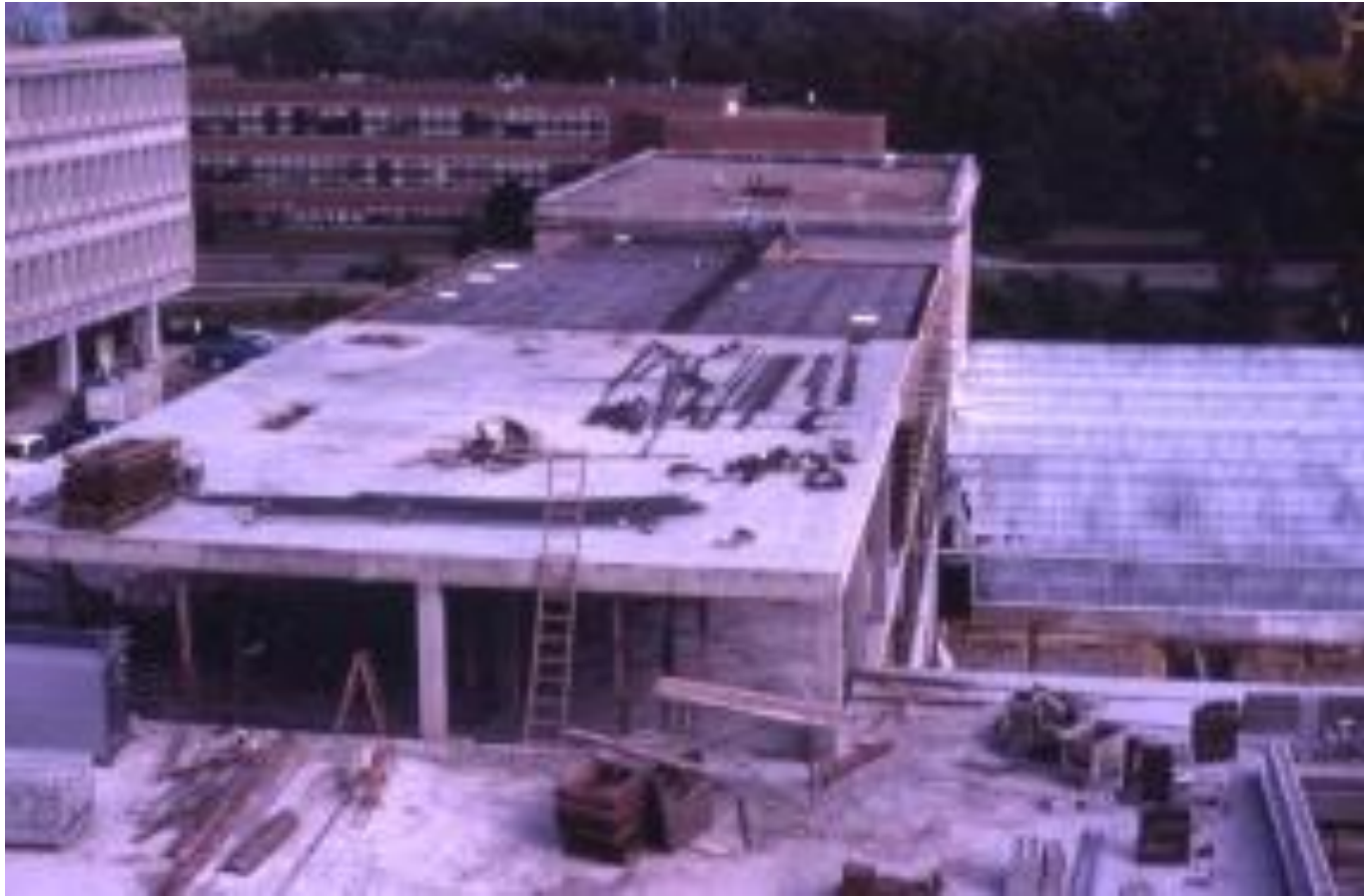
Construction of the second floor.
