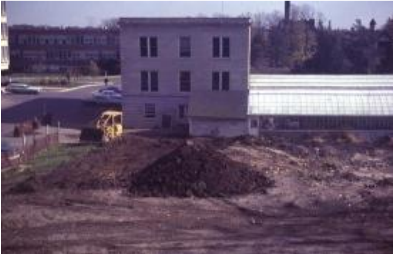
Preparing the site.
