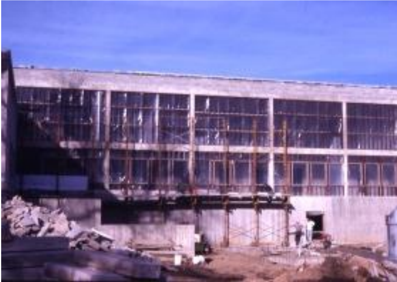
The addition during construction as viewed from the south.
