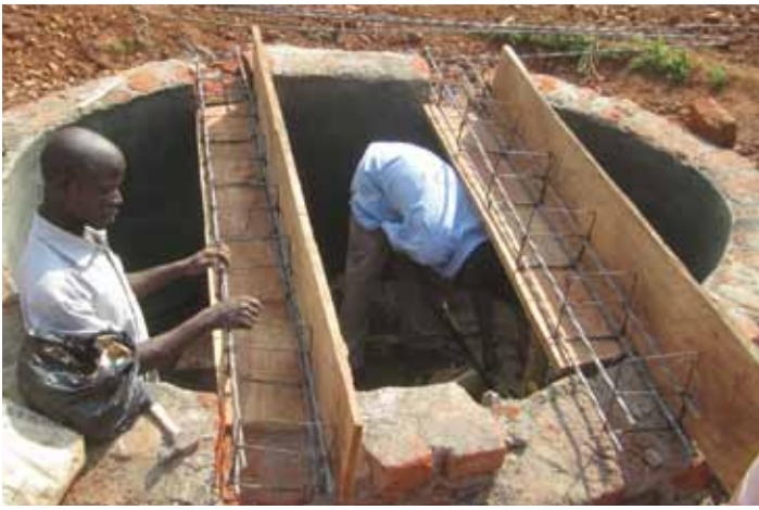
Building a cistern for run-off from the school's deep well.
