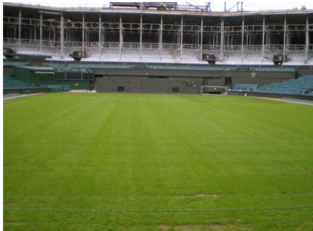
Centre Court on August 15 after renovations.
